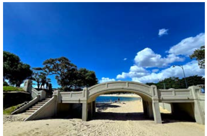
Day 4: Rocky Point Island Bridge at Balmoral Beach
